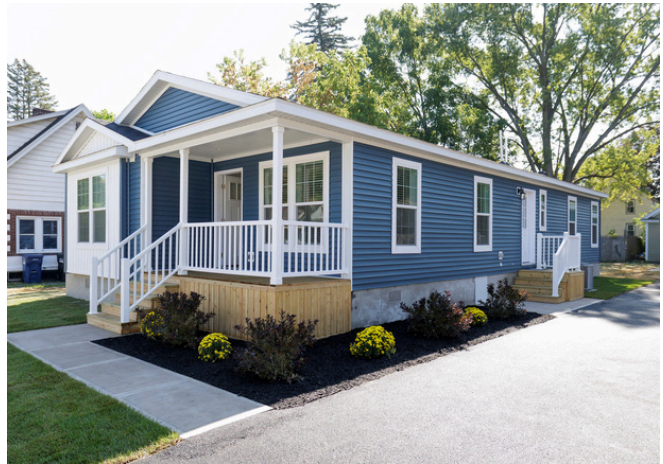
Left: A modular home in Syracuse built through the MOVE-IN NY program. Photo courtesy of the State of New York.
