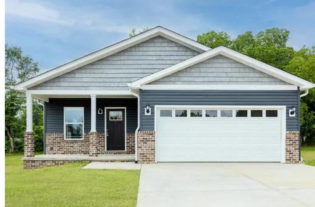
Example of a CrossMod, which could be applicable to the Ski Lodge site.
