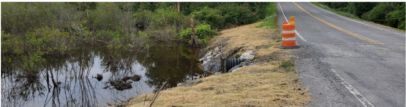
POWERS, S. 2024. ROAD-STREAM CROSSING NEW LEBANON, NY
