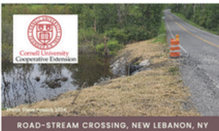
ROAD-STREAM CROSSING, NEW LEBANON, NY
