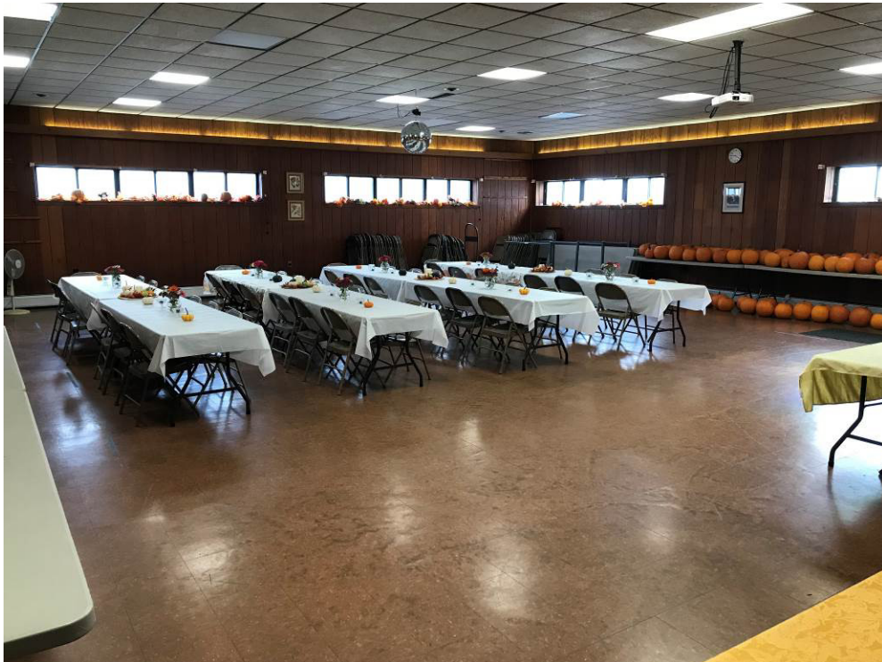
Red 12" Floor Tile in Social Hall
