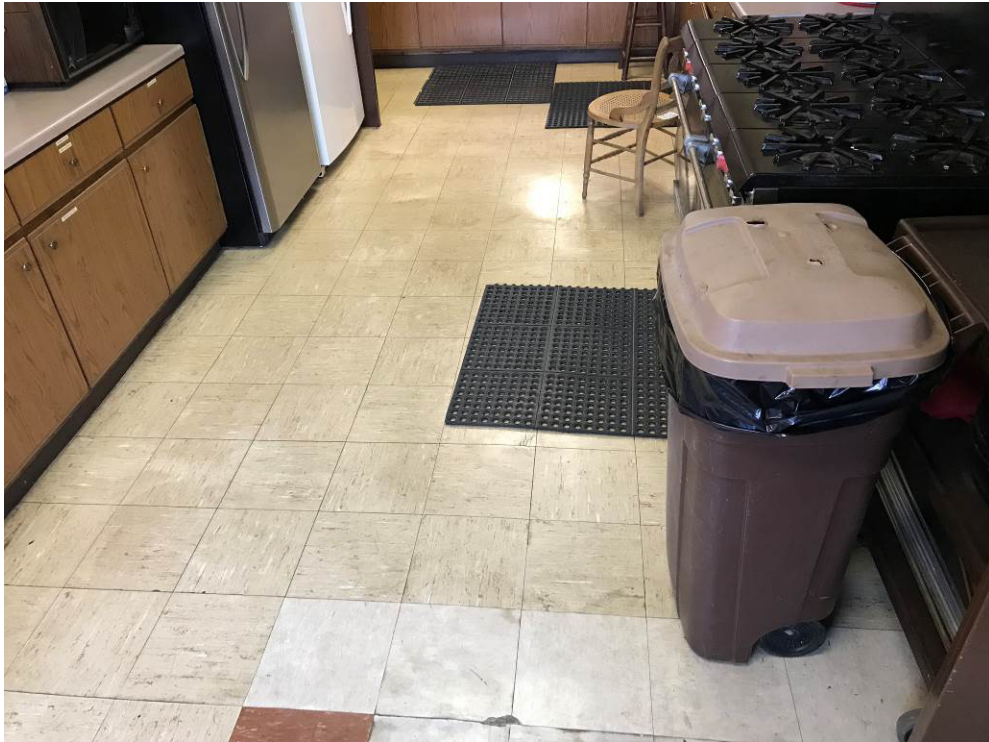
12" Floor Tile in Kitchen
