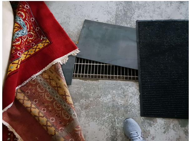
Photo 15: Floor Drain in Firefighting Vehicle Bay
