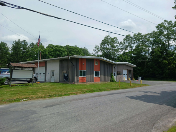
Photo 4: Right Elevation with Partial Front Elevation
